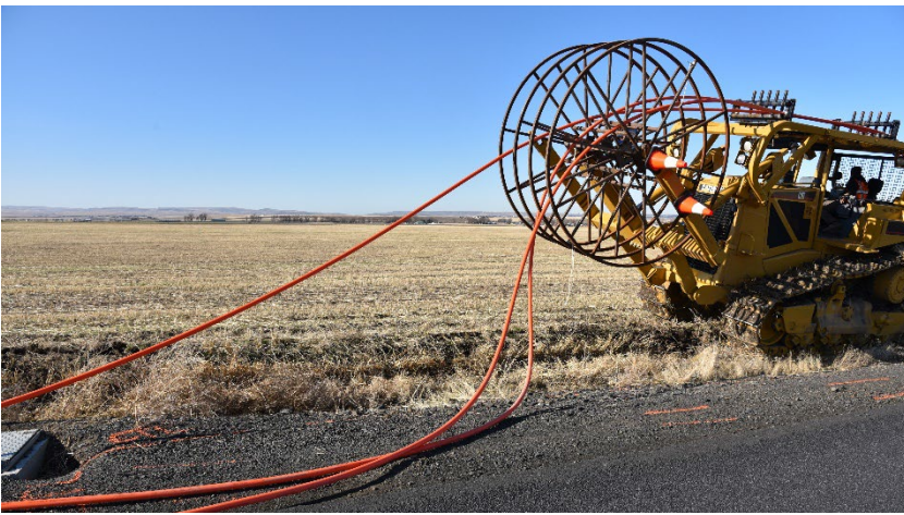
CBP Fiber Optic Cable Installation, CTUIR
