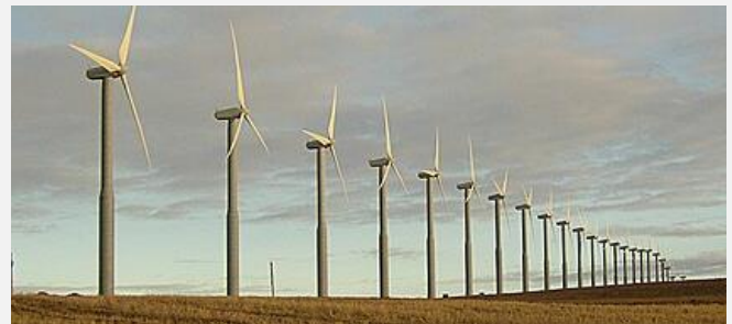
Staterline Wind Farm
